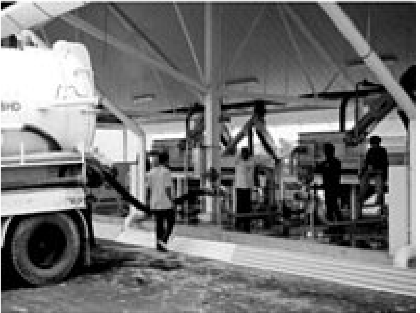
Tanker delivering septic sludge into the HUBER ROTAMAT® Sludge Acceptance Plant Ro 3.3
