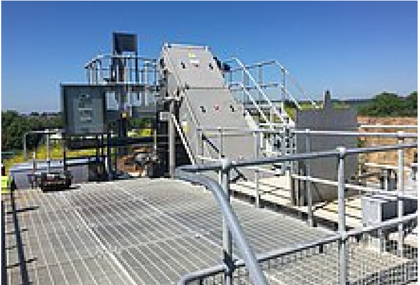
New RakeMax® screen installed on top of the existing balance tank
