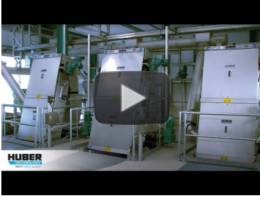
Video: HUBER Coanda Grit Washing Plant RoSF at a municipal WWTP https://www.youtube.com/watch?v=SH3P8IpCDJM
