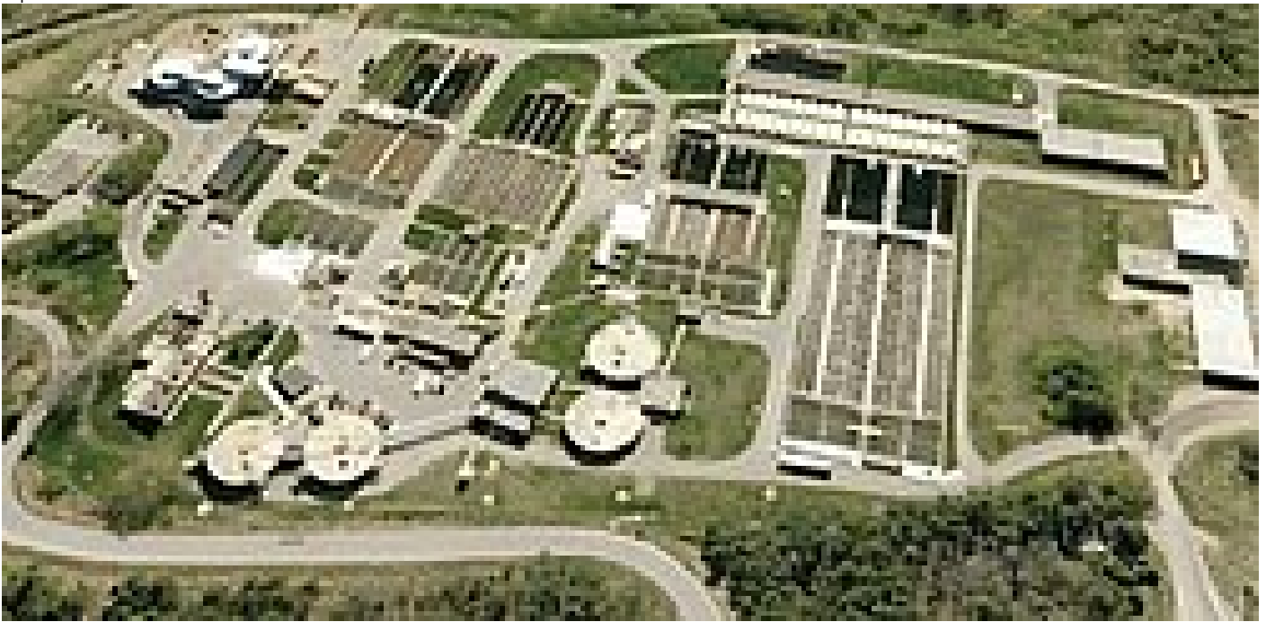
Aerial view of Gulph's treatment plant
